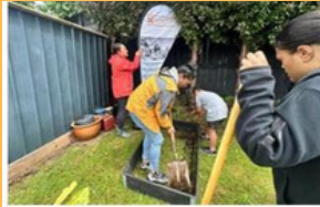
Marking out the garden area
